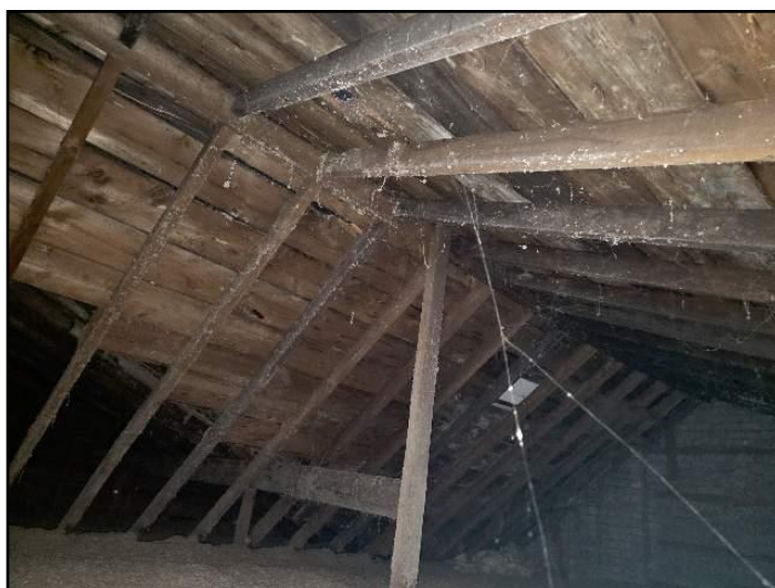
14. Rafters/ceiling joists
