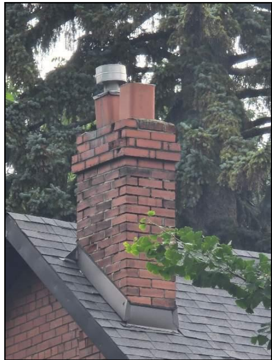
30. Inspect chimney, and sweep, if needed be
