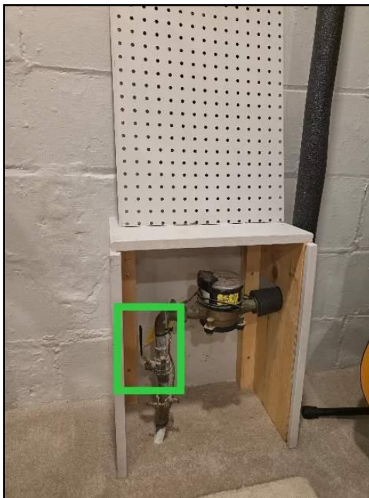
34. Front of the basement
