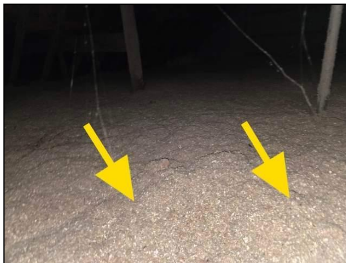
33. Amount less than current standards
