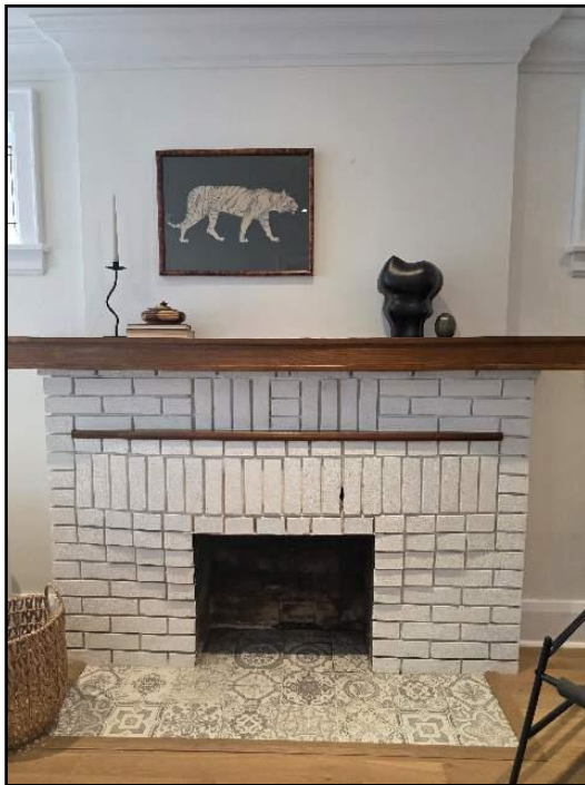
29. Inspect chimney, and sweep, if needed be
